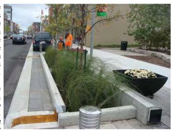
Streetscape improvements should also be designed with stormwater management in mind. Pervious brick pavers are now available. Also, brick pavers can be installed without the use of mortar, which reduces runoff and also allows easier removal and reinstallation when underground utilities need repair. Where the main pedestrian pathway is constructed of concrete, un-mortared pavers can be used between the main sidewalk and the curb, and between the main sidewalk and a building.
