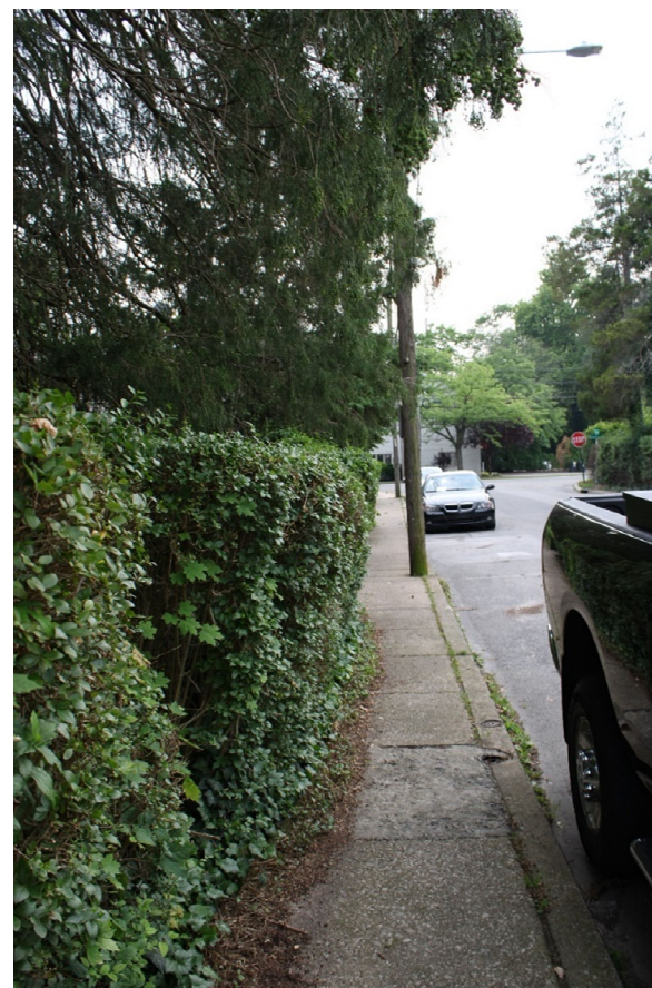
Figure 21: Vegetative encroachment on the sidewalk. Photo credit: CHPlanning
