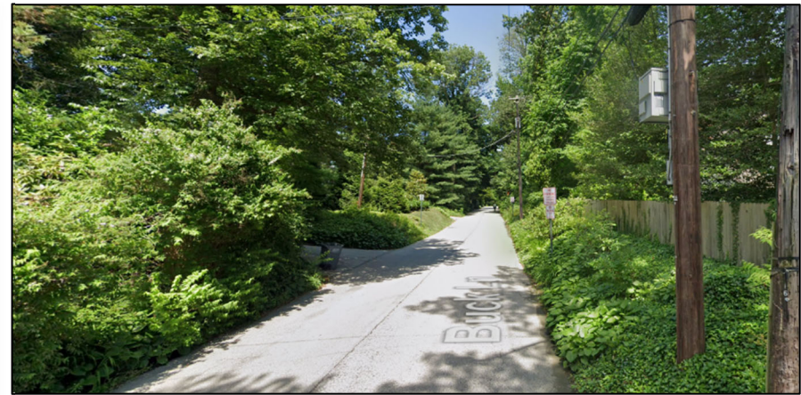
Figure 14: Current Condition of Buck Lane
