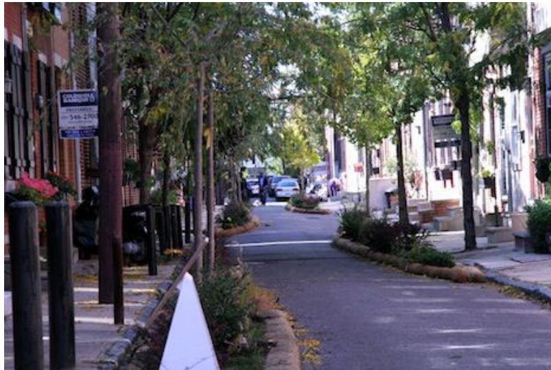
Figure 25: Vegetated chicane on tree-lined street
