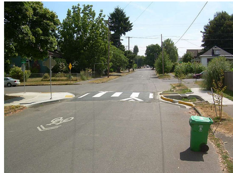
Figure 22: Raised crosswalk with curb extension to narrow the entrance to residential streets
