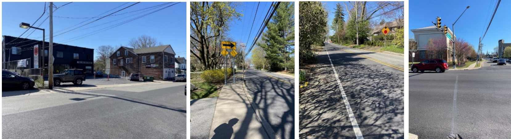
Figure 10. High Risk Road Features in the Brynford Neighborhood
