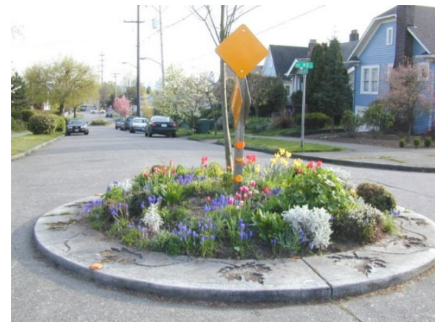
Figure 18: Example of a mini roundabout with plantings and decorative imprints on the concrete curb. Source: Bicycle Safety Guide and Countermeasure Selection System (pedbikesafe.org)
