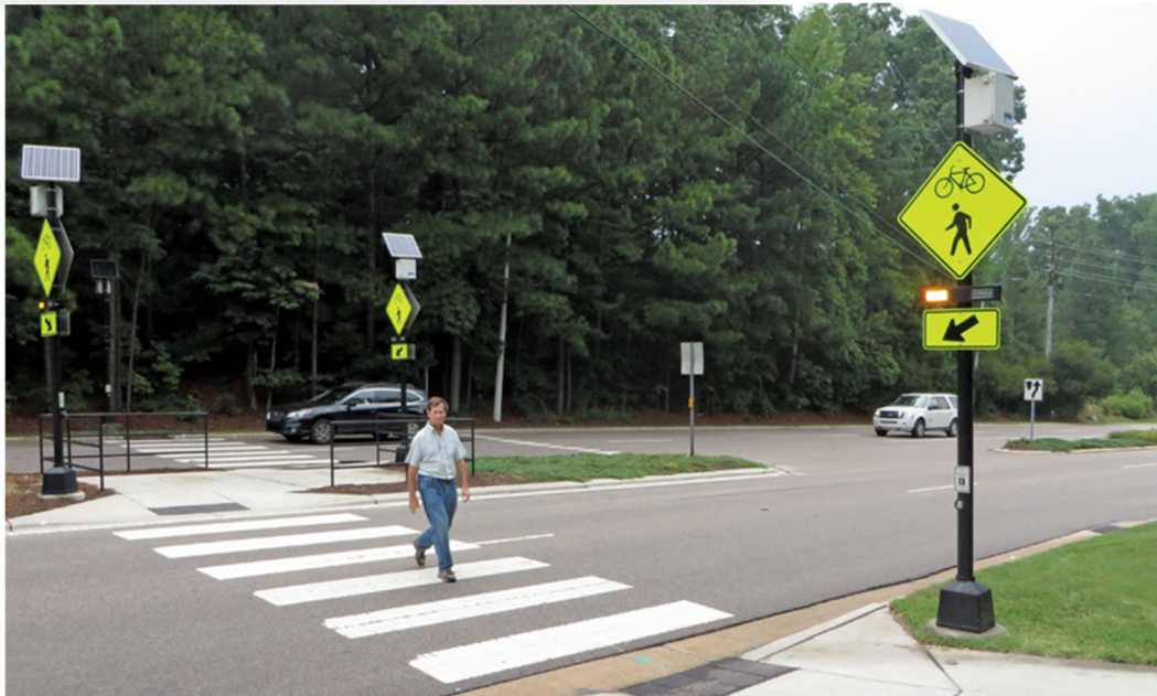
Figure 20: Example of Rapid-Flashing Beacon Pedestrian Crossings. Source: New Rapid-Flashing Beacon Shows Great Promise in Improving Pedestrian Safety — Center for Transportation Safety (tamu.edu)
